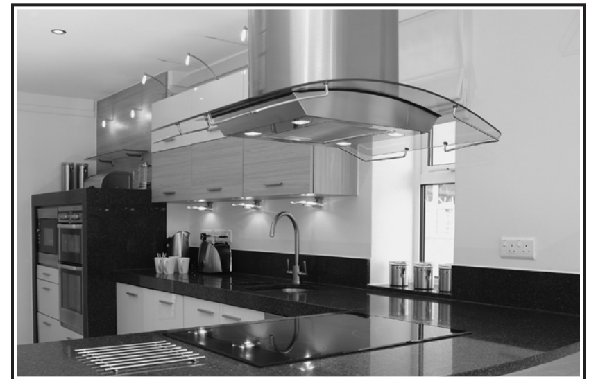
An example of a chimney-style hood over a peninsula. These hoods are 27"-30" deep. I wouldn't recommend this arch for someone tall unless we set the install height from the lowest points on the curve.
